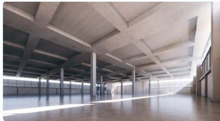
3D Model: Design of Prestressed Concrete Flooring Structure
