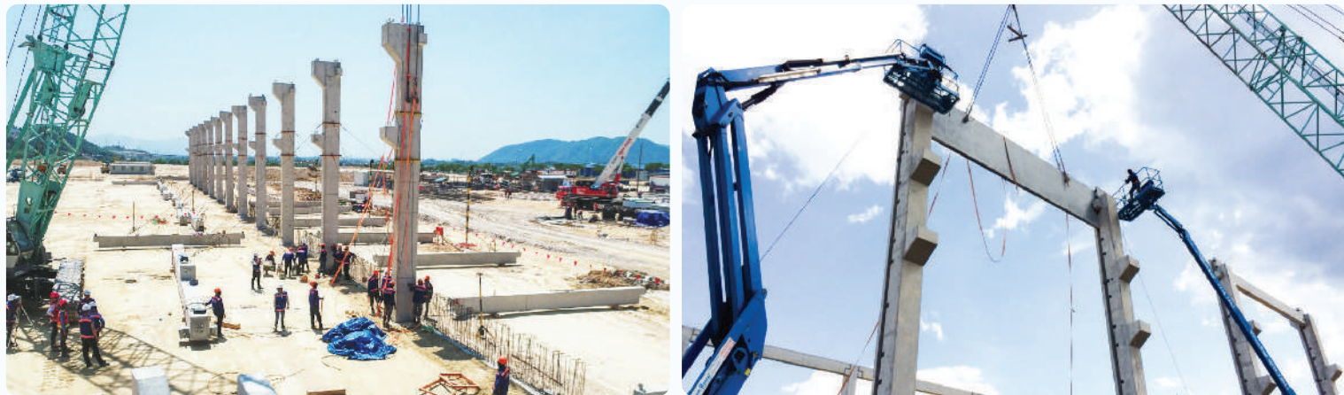
ERECTION OF PRECAST CONCRETE COLUMNS, WALL PANELS
